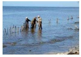
Figure 3. Palisades established to reduce wave force and promote red mangrove establishment and growth.
